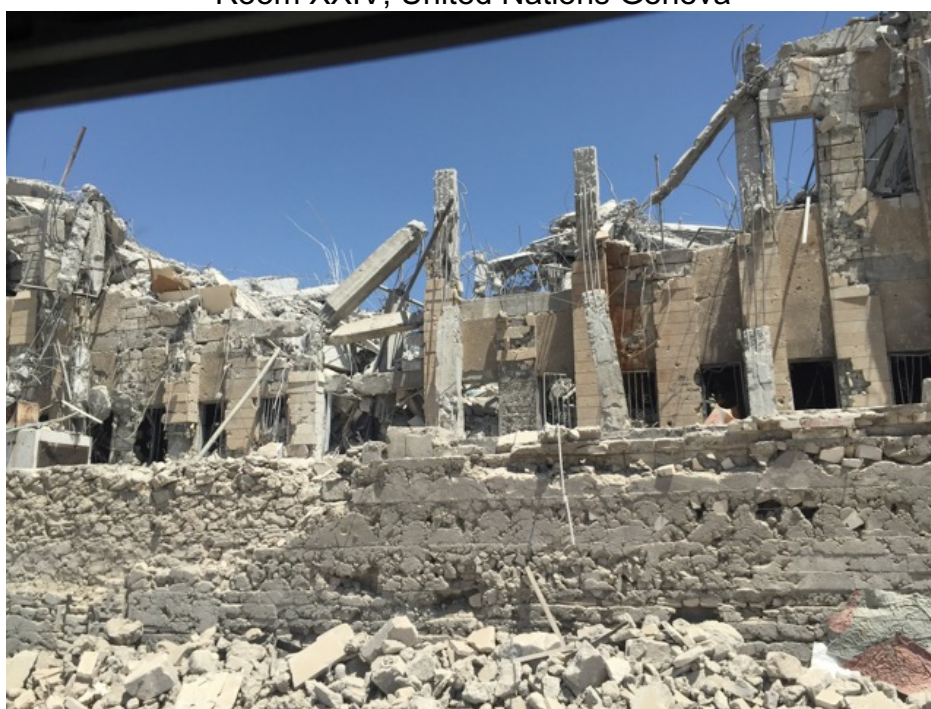
Damaged buildings from the use of a bazooka in West Mosul, Iraq. August 2017. © Sahr Muhammedally, CIVIC
