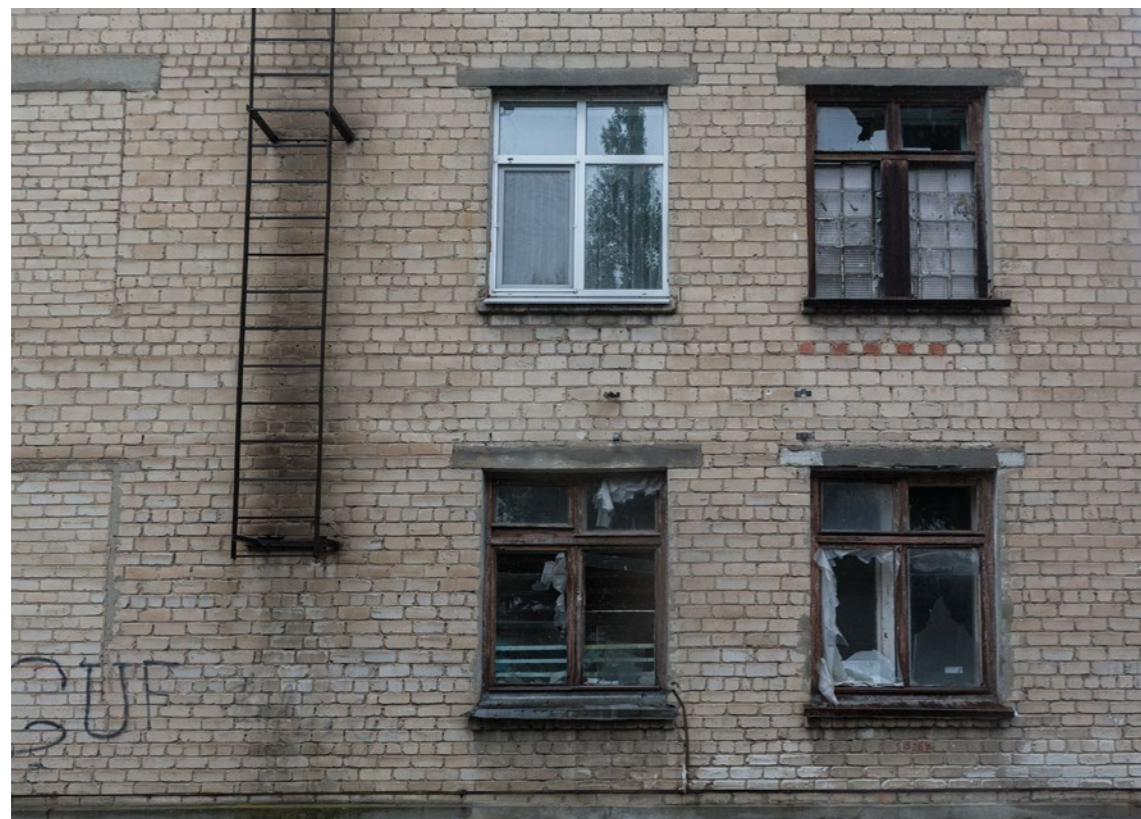
Explosive weapons shattered windows at Maryinka District Central Hospital in Krasnohorivka. While some windows had been replaced by September 2016, others consisted of broken glass and torn plastic sheeting. © Anton Skyba for International Human Rights Clinic at Harvard Law School and PAX / September 2016.
