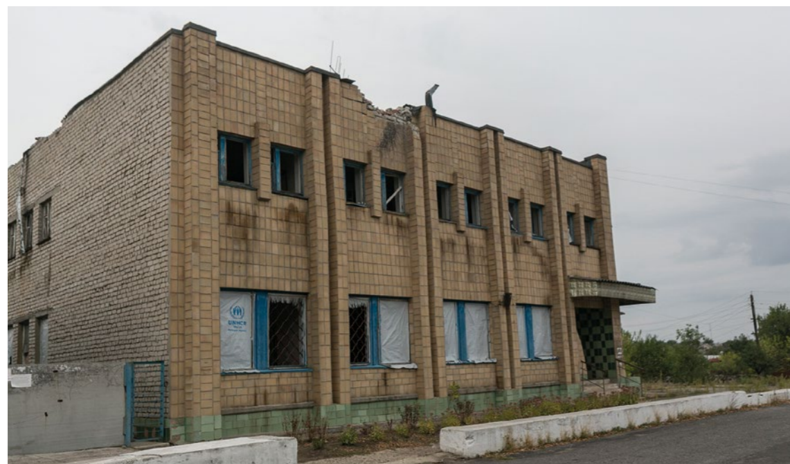
Explosive weapons knocked out Granitne's telephone station, located in the town post office, on one of the first days of the armed conflict. The loss of the station made it more difficult for residents to communicate with the hospital or ambulance station. © Anton Skyba for International Human Rights Clinic at Harvard Law School and PAX / September 2016.
