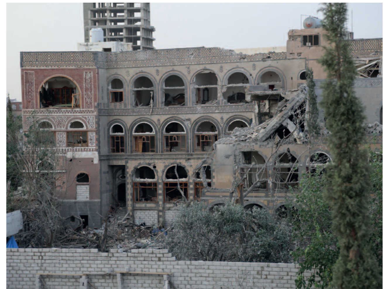
Houses damaged by shelling next to Sabaeen hospital in Sana’a on 15 June 2015 (OCHA/Charlotte Cans, 7 July 2015)
