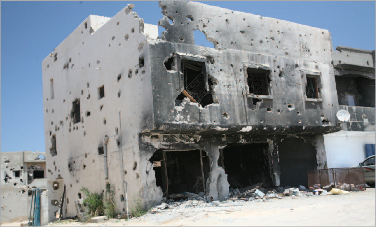
Shop fronts in Sirte, showing the long-term damage from both the blast and fragmentation effects of explosive weapons.
