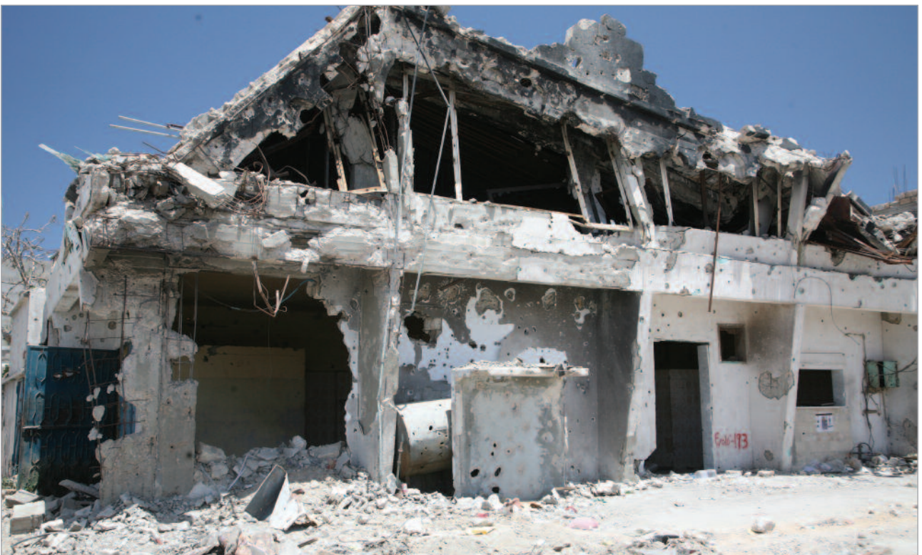
Shop fronts in Sirte, showing the long-term damage from both the blast and fragmentation effects of explosive weapons.
